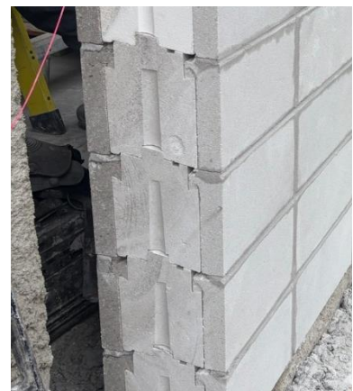
Example of insulation overlap and continuity.
