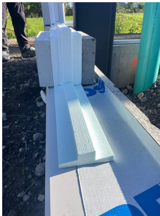
Example of starting block assembly
